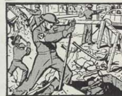
ROAD REPAIR CREW
